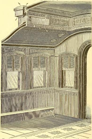
Showing a corner of car at opposite end from the heater, with termination of hot air pipe on one side and deflecting orifice for the fresh air; also, one of the exhaust pipes and weather caps, at top, for the removal of vitiated air. NEW,
